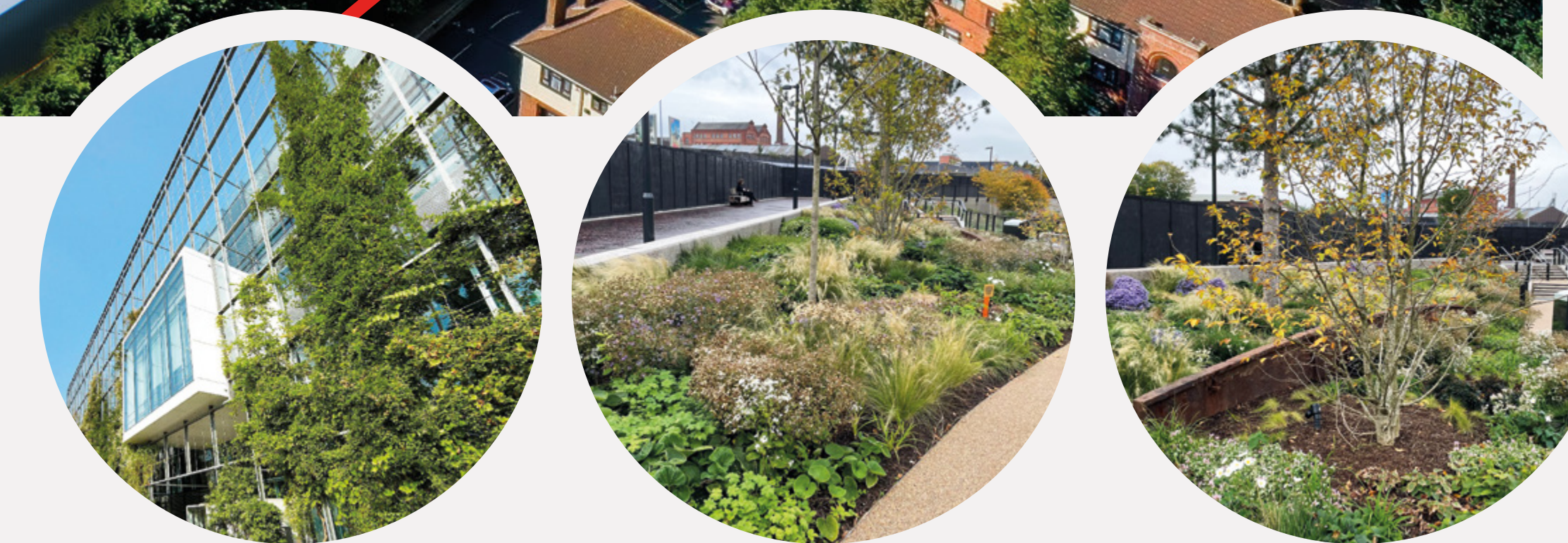
Public realm and landscape improvements proposed as part of the Phase 1 development
